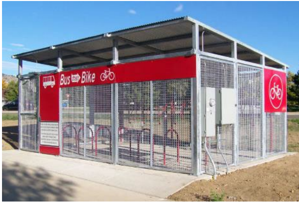
Gated Shelter and Rack
