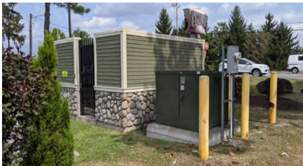
Figure 27. Screening of mechanical equipment.
