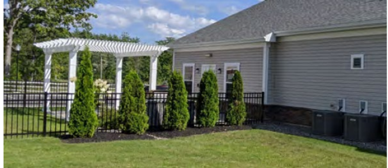
Figure 25. Screening of mechanical equipment.
