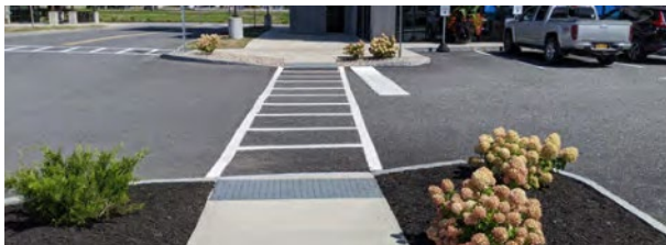
Figure 17 Internal parking lot crosswalk.
