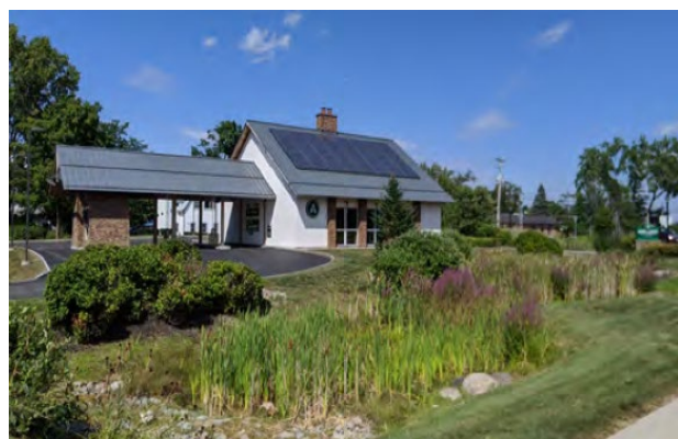
Figure 24. Stormwater retention pond at a commercial bank designed to look like a natural area.
