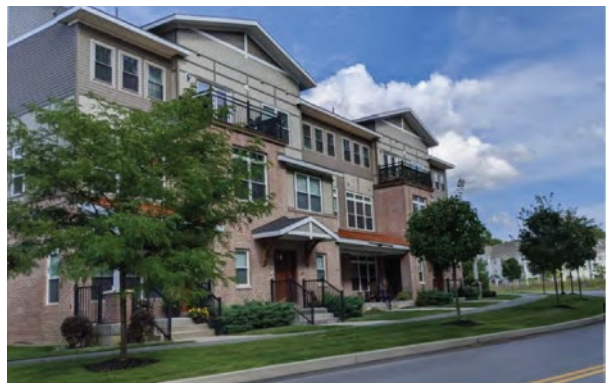
Figure 31. Building massing. This long building is nicely broken up with strong depth fluctuations in the facade and roofline which help to identify individual apartment entrances and create balconies.
