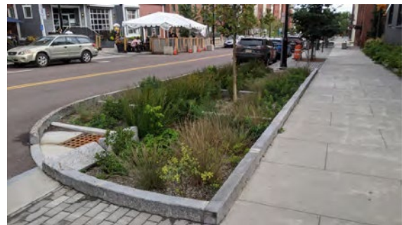
Figure 21. Stormwater retention with rain garden.
