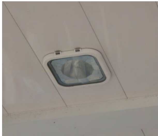
Figure 36. Gas station canopy light. This recessed light in a gas station canopy is ideal because it focuses the light downward and reduces glare to passing motorists.
