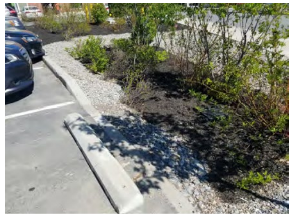
Figure 19. Stormwater retention. Use of creative stormwater retention designs can allow for landscaped areas to absorb rainwater locally and filter it without it having to be piped underground, where it can pollute the local waterways. This design has a lowered curb edge which allows the rainwater to flow down into the lowered planting bed where it can be absorbed by the ground and provides water for the plants. A hidden overflow pipe allows excess water to escape to prevent overflow.
