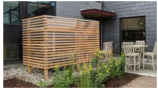
Figure 28. Screening of mechanical equipment.
